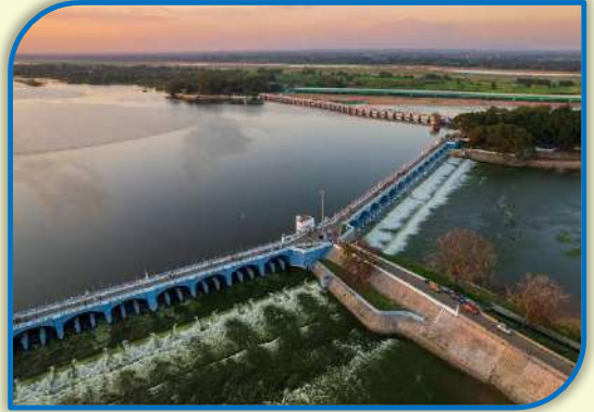
Kallanai Dam 68.2 km from DSAC
